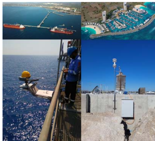
Figure 1 Monitoring system in Vasiliko VTTV (left) and Ayia Napa Marina (right), Cyprus
