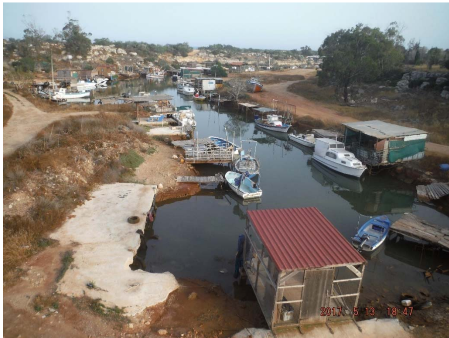
Photo 3. Structures made from local fishermen on the riverbanks had to be removed by hand and light machinery
