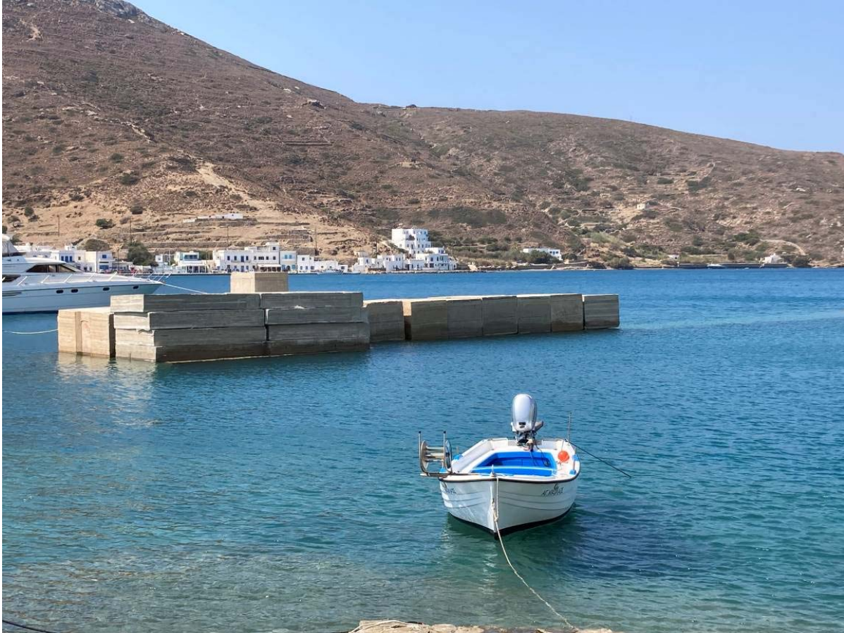
Photo 4. The fishing shelter's breakwater head, was built using the existed cellular artificial blocks
