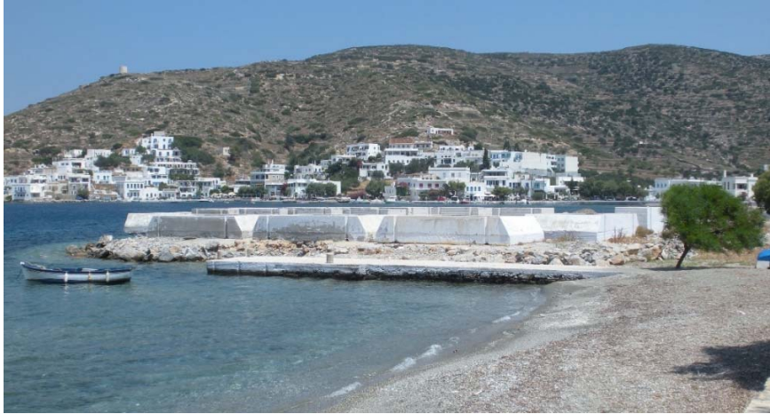
Photo 1. Katapola beach (2015) shortened by the pier, consisted of embankment material and 17 concrete blocks
