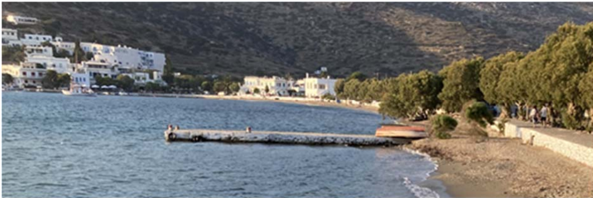
Photo 8. After the construction of the shelter, Katapola beach has been freed and rebounded (2022)
