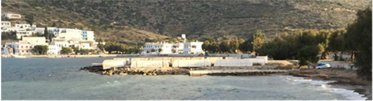
Photo 7. Old concrete materials were forming a pier perpendicular to Katapola beach (2015)
