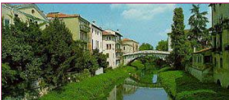
One of the bridges on Retrone River ( www.comune.vicenza.it )
