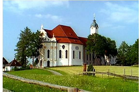
Total view of Wieskirche Church
