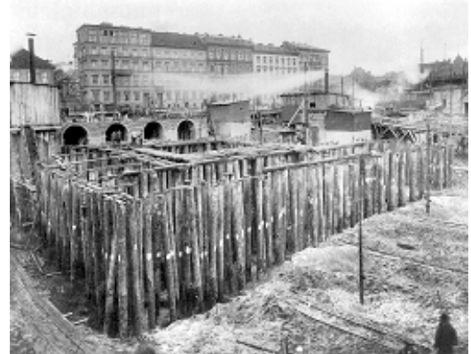
Pile foundation of 1912
