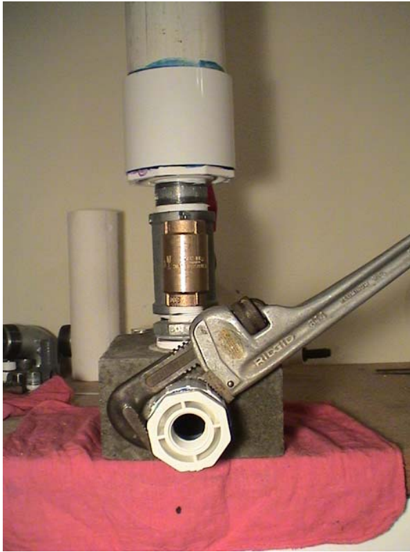
Installing the 2" to 1" PVC Bushing
