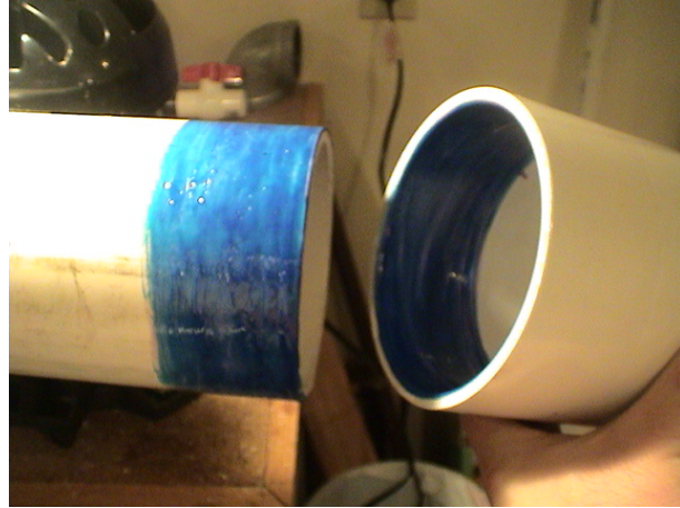
Pipe and Coupling with PVC Cement
