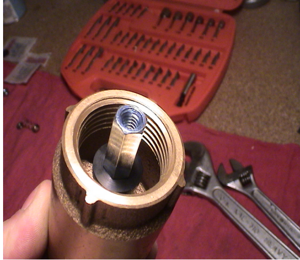
Faucet Washer and Coupling Nut installed.
