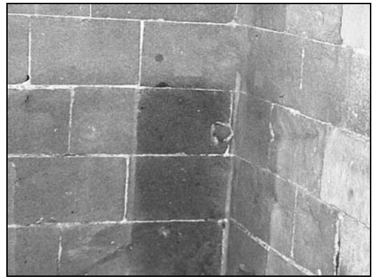
Figure 10. The calcarenite blocks where the measurements of Figures 8 & 9 were performed.
