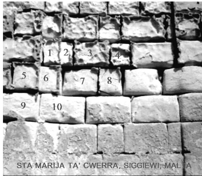
Figure 6. Apart of the external southern wall of the church. Numbers correspond the points of measurements.
