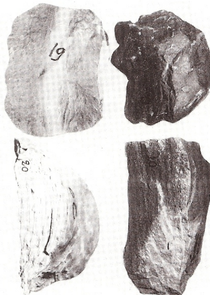
Fig. 6 : Building stone samples showing a zonal weathering. 8, 10 : Sandstones; 19 : Limestones; 20 : secondary calcite which cover building stones.
