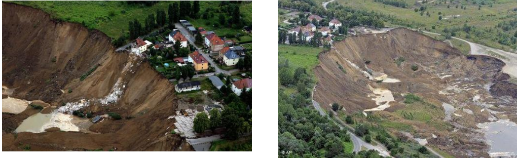
Fig. 1. The landslide of July 19, 2009, in Nachterstedt (Petley, 2009, http://daveslandslideblog.blogspot.com/ )
