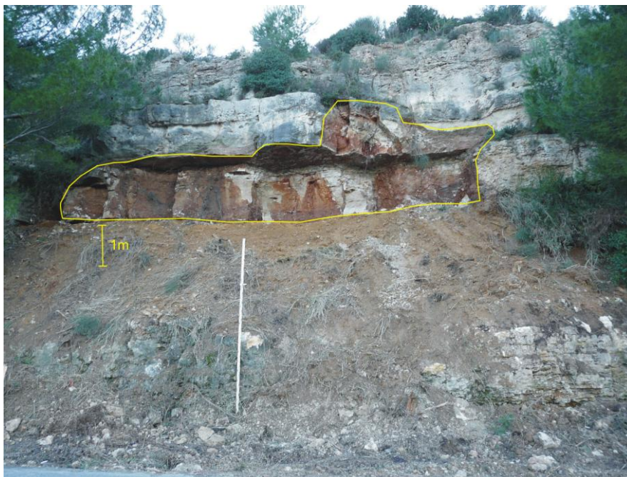
Fig 3. Source area of the rock falls occurred on December 16, 2009.
