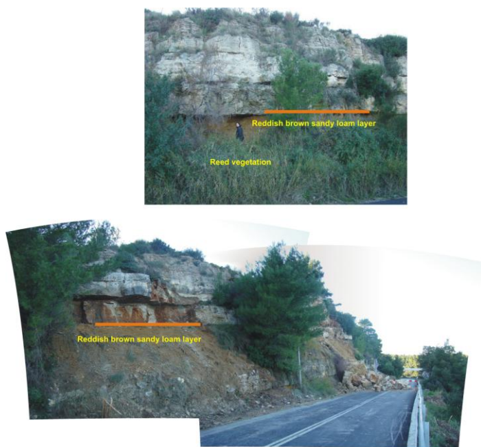
Fig 7. The layer of reddish-brown sandy loam is slowly washed out by the percolating water from the overlying limestone (note the beginning of undercutting). The water favors thick reed vegetation. It is a matter of time this slow process to undercut the limestone causing a rockfall in this place in the future.
