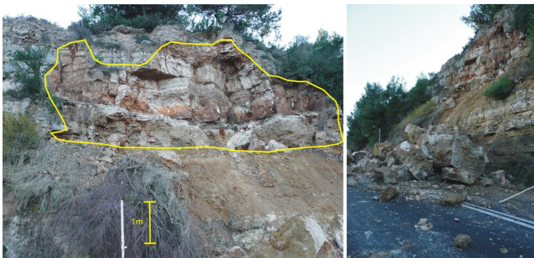
Fig 4. Source area of the December 21, 2009 rock falls.
